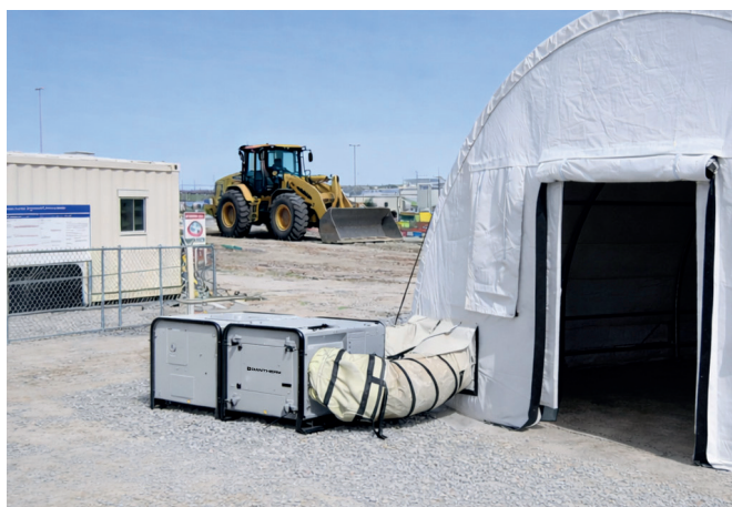
Installation with the air ducts
