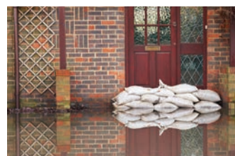
Water Damage Restoration
